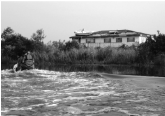
Members of Prattville’s swift water rescue team search for survivors in Mississippi and witness Katrina’s haphazard deposition of debris. Notice the boat resting on top of the house in this picture.
